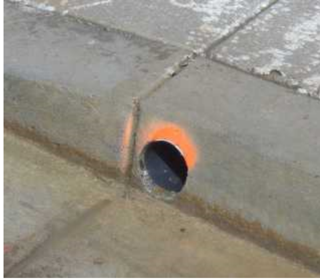
Figure 2.3.2 – Typical Roof Drain Curb Outlet at Sidewalk
