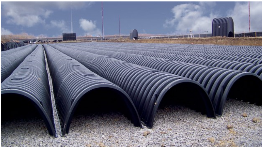
Figure 2.3.3 – Typical Underground Infiltration Chambers
